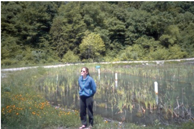
Figure 11. The upper surface of a vertical flow system constructed in 1990 to receive effluent from Westmoreland Coal Company's Pine Branch refuse pile (Duddlestone et al. 1992). The vertical plastic piping visible in the background was installed to enable "clean out" of the drainage system, should that prove necessary, prior to the development of the flushing valve concept depicted in Figure 13.
