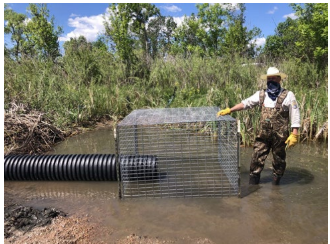
Figure 10. Example of a derivation of the Beaver Deceiver flow device. (Photo, “Beaver Deceiver,” 2020, by Alex Schubert of the U.S. Fish and Wildlife Service Mountain Prairie, is online at https://www.flickr.com/photos/51986662@N05/50091655076 .)
